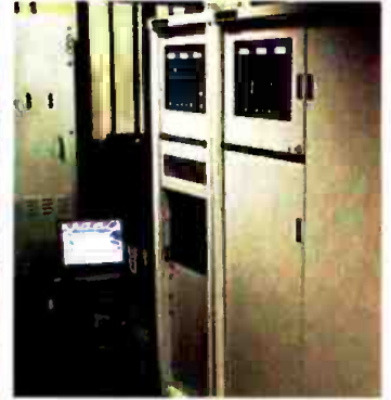
wsb-tv has a new all-digital studio. The station's Harris DTV 100 kw transmitter is outfitted with an ATSC-compliant encoder.
